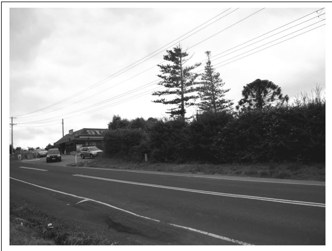
A section of the hedgerows trimmed in 2006 (6 years ago), looking good but now ready for a heavier one metre high trim. Note erosion gully on nearside verge, far deeper on both sides of the road further southward.
