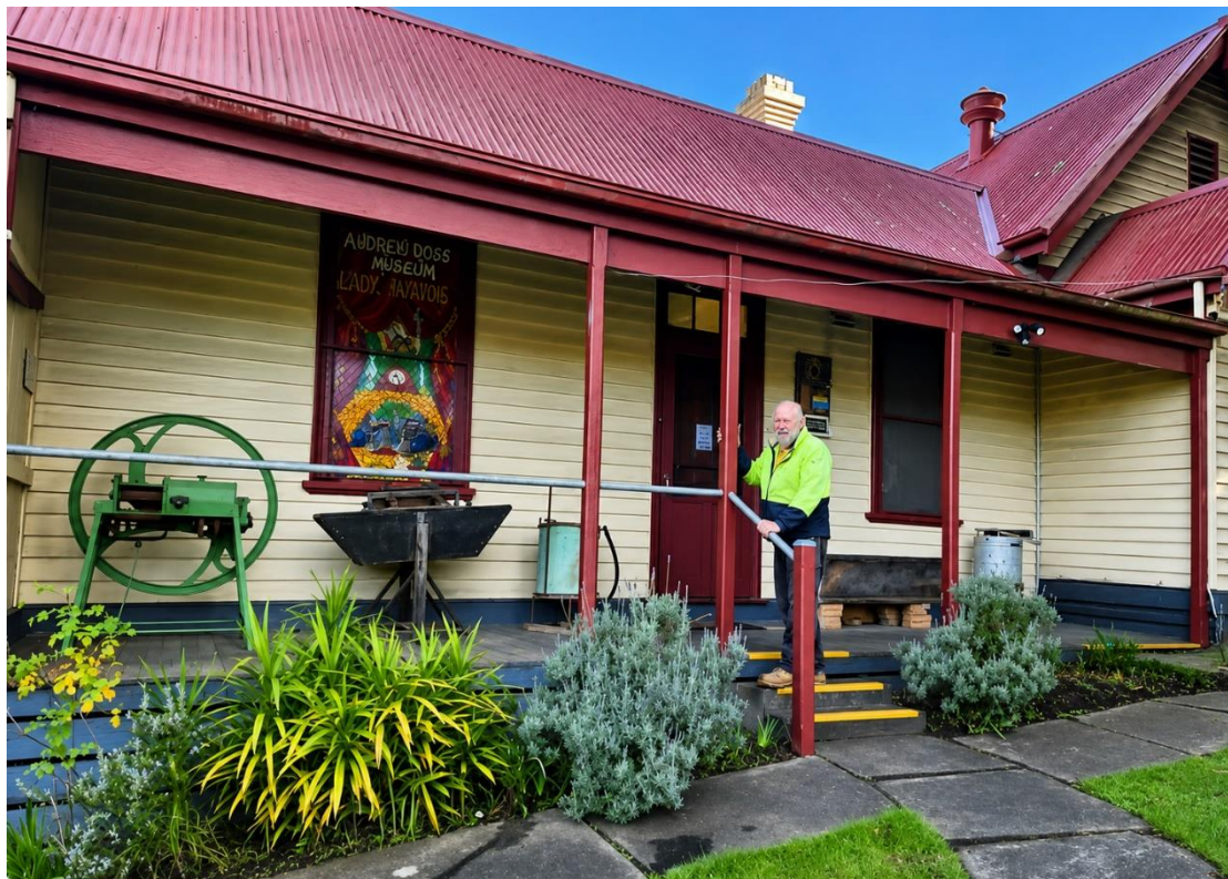
Brendan McOrrie inspecting the newly installed safety rails.
